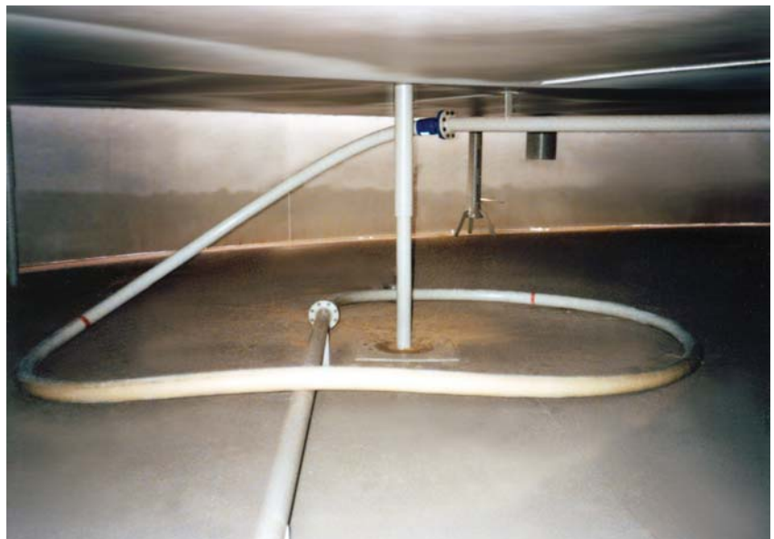
Installed Drain Pipe System
